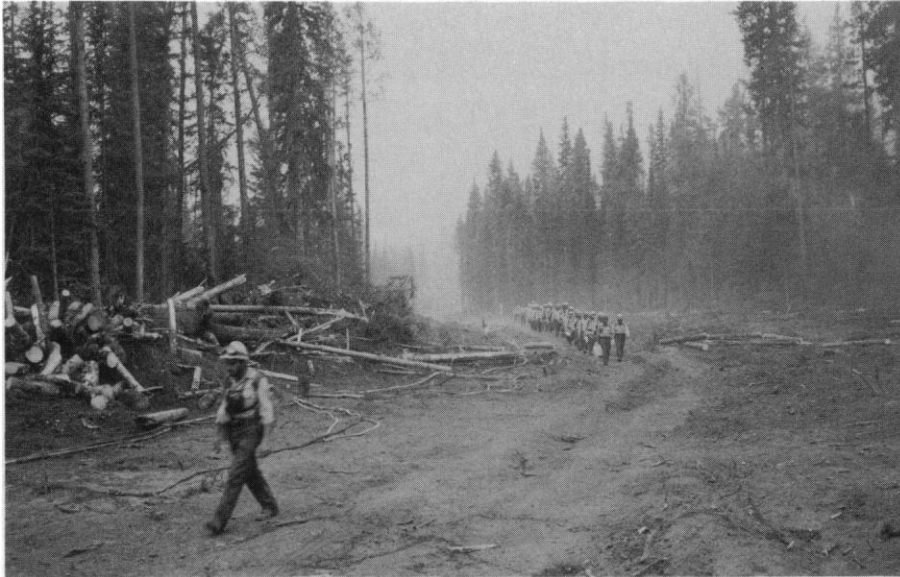
Figure 4. Bulldozers were used to cut fire lines, in this case in Gallatin National Forest near the northeast entrance to Yellowstone National Park and to Cooke City, MT. Fire fighters are moving through a bulldozer-cleared area where all trees have been removed for a width of at least 8 bulldozer blades. Bulldozer lines proved no more effective than hand-dug lines at holding fast-moving fires and left scars that will remain indefinitely. Photo: Jim Peaco, National Park Service.
